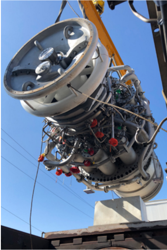
Installation of the new thermal block onsite.
